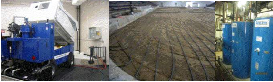
Pictures from left to right: snow melt pit, subflooring heating, preheating water
